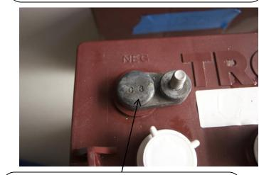
Trojan stamps the date the battery was made into the top of the negative post. The letter represents the month and the number equals the year. This battery was made in March of 2003
